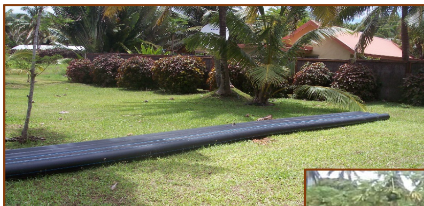
Pipes stored incorrectly at Aroa placed on the ground instead of being placed in timber cradles
